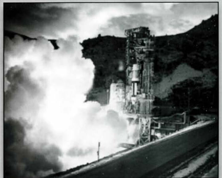
A Titan first stage is tested at the Waterton Canyon, Colorado, Martin plant (Lockheed/Martin photo).
