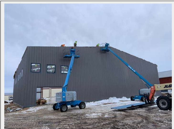
New Spirit of Flight building under constructed in Nampa, ID
